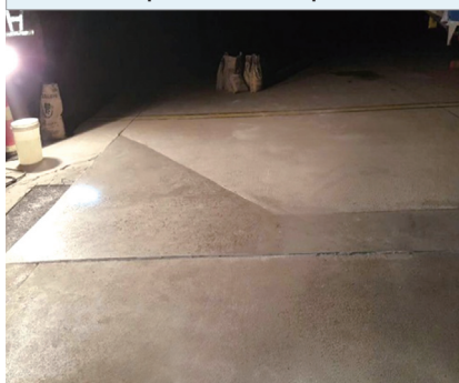
Airport floor repair
