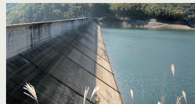
Sancheong Pumped-storage Plant
