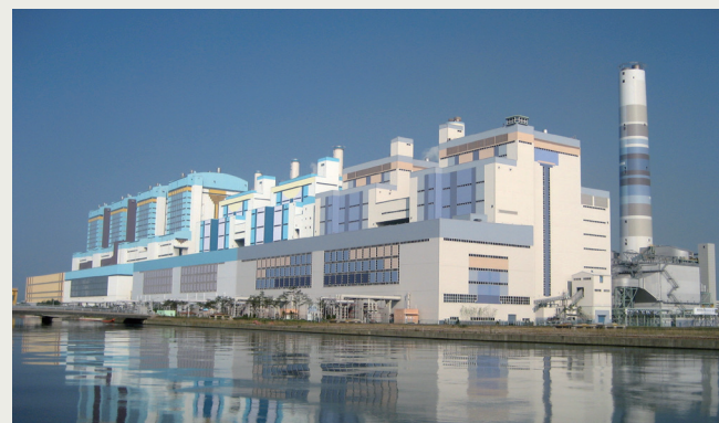
Taeon Power Plant
