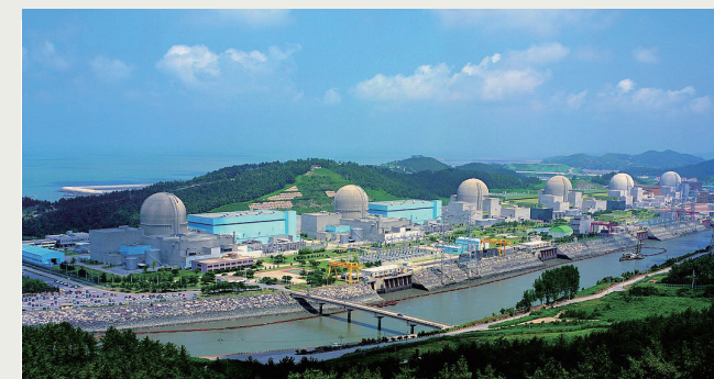
Hanbit Nuclear Power Plant
