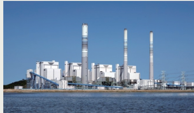
Yeongheung Power Plant
