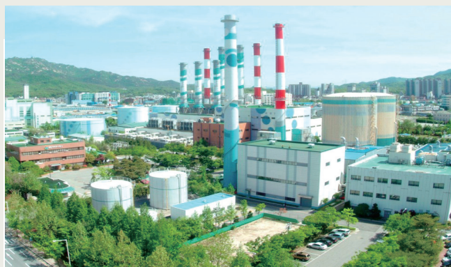
Pyeongtaek Power Plant
