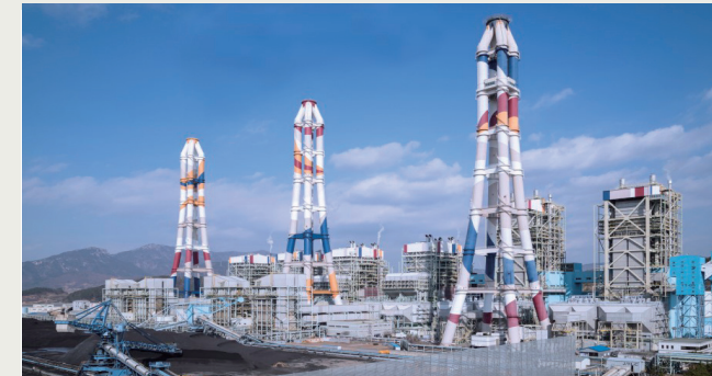
Samcheonpo Power Plant
