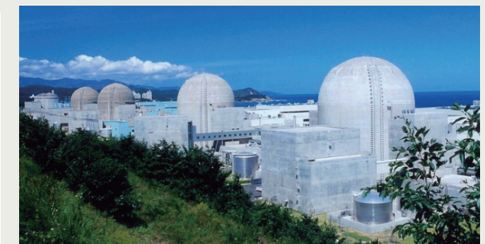
Hanul Nuclear Power Plant
