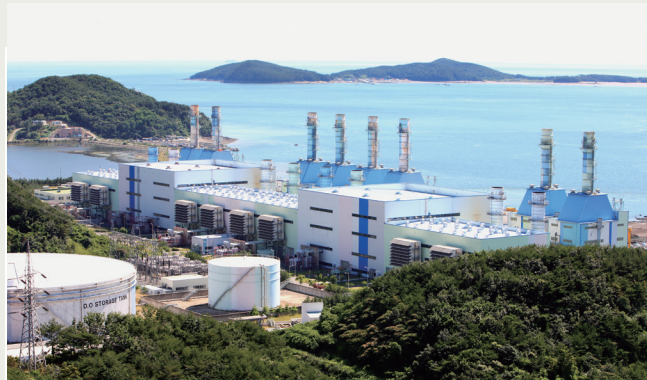
Boryeong Power Plant
