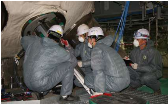
Eddy Current Test for SG Tubes
